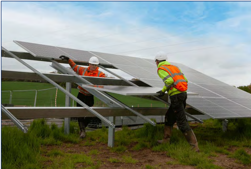
Plate 12-24 PV module installation (Ref. 12-16)
