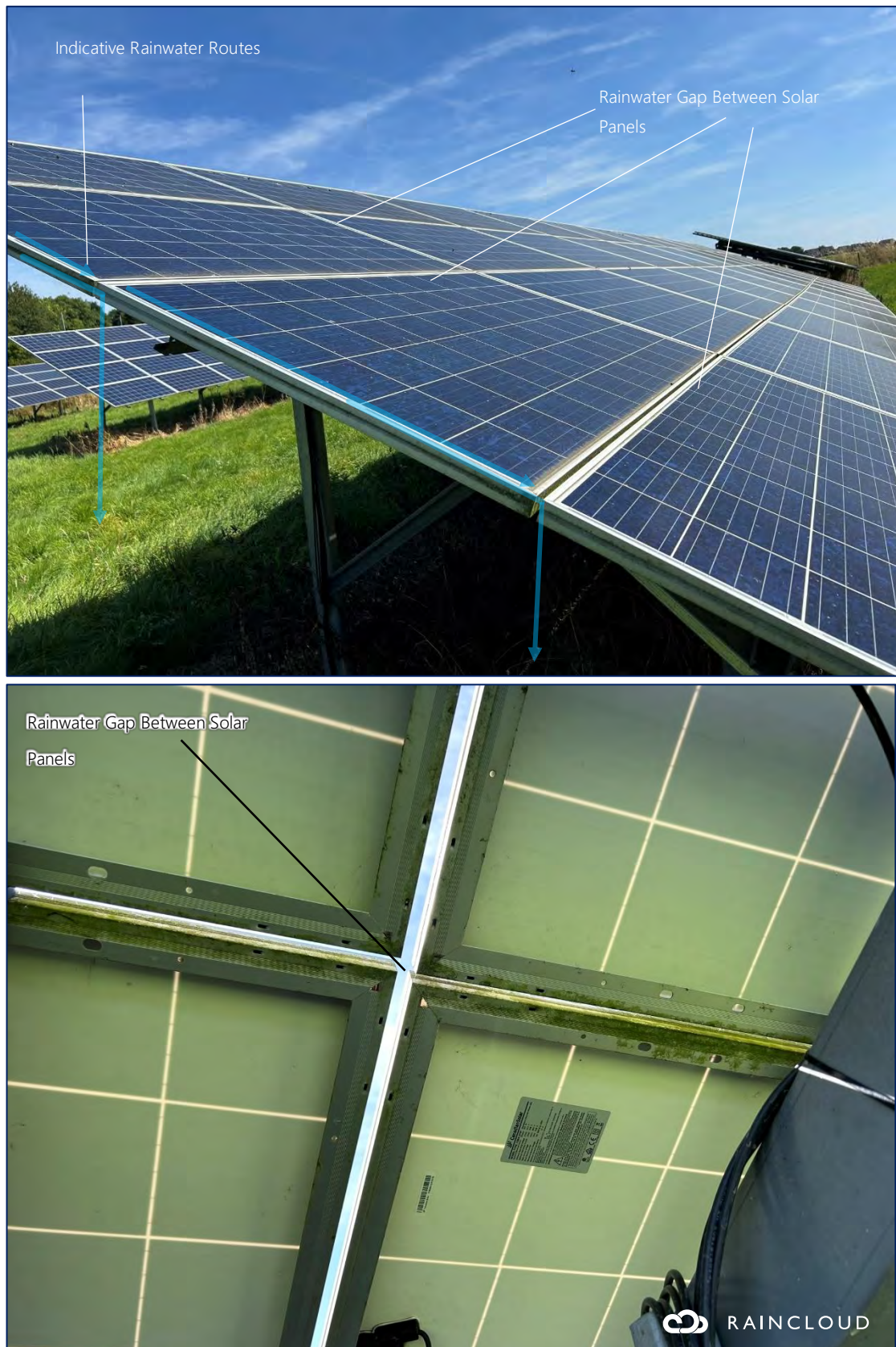
Plate 12-25 Rainwater gaps on PV array table
